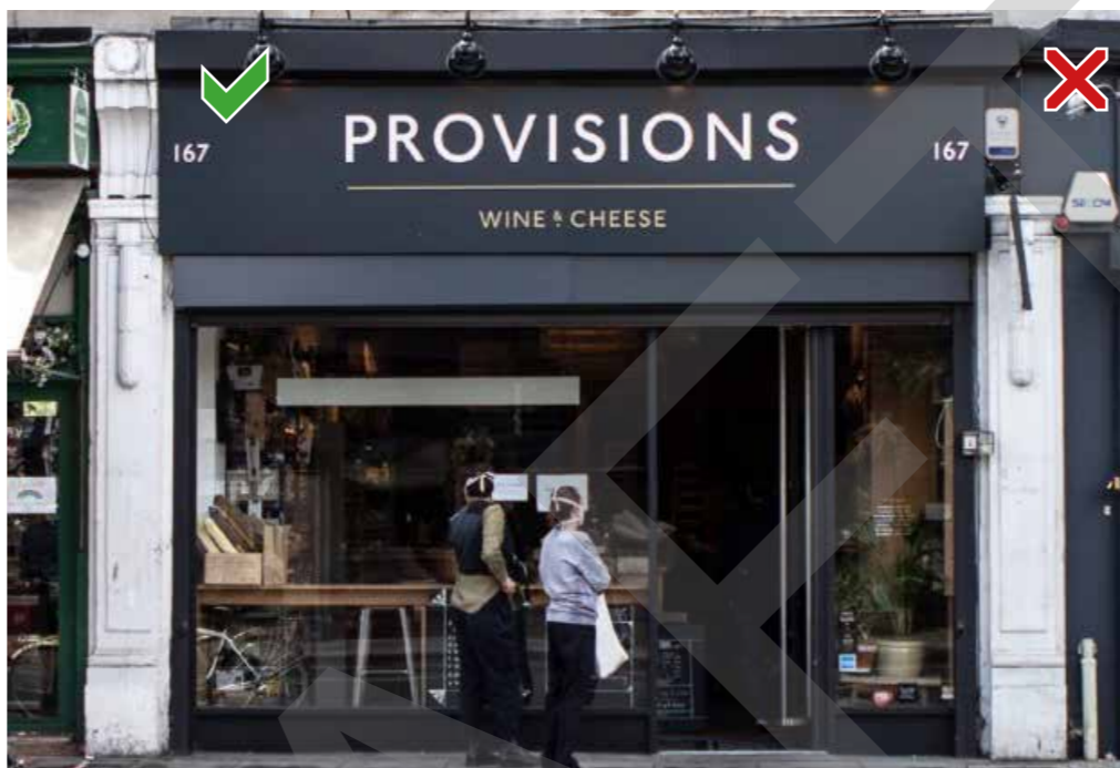
Treatment of original pilasters intended to separate shop fronts varying within adjacent shop frontages dependent upon which shop owner takes responsibility for the architectural element. The detail, if intact, should remain visible and not hidden in favour of bland over boarding matching inappropriate fascias.
