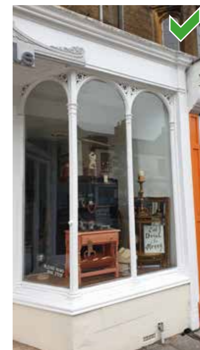
Carved timber mullions introducing vertical lights, shadow producing depth to the frame
