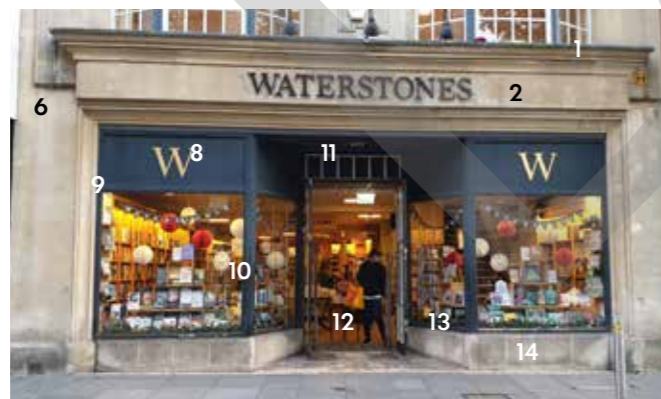
Left: Late 20 th century interpretation of the shop front Employing original intent, pilasters insinuated with a string detail, incorporating the cornice and fascia in stone within the elevation.
