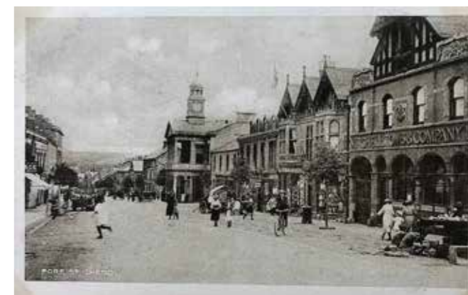
Fore Street, 1900 New builds to the east of the Post Office
