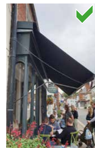
Blind box installed above cornice and fascia
