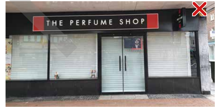
Internal grilles set behind glazing, that disallow visual access - less desirable
