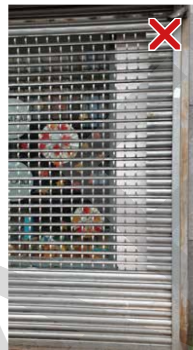
Grille protecting stall riser, allowing visual clarity, preferable to solid full depth grilles, though not desirable
