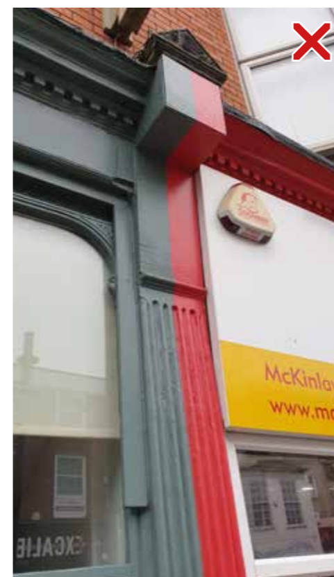
Treatment of original pilasters intended to separate shop fronts varying within adjacent shop frontages dependent upon which shop owner takes responsibility for the architectural element. The detail, if intact, should remain visible and not hidden in favour of bland over boarding matching inappropriate fascias.
