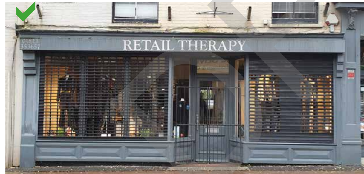
External security grilles set within the window frontage of a Grade II listed building, allowing visual access to shop window combined with successful way of securing a recessed entrance. The shop signage and fascia extends down in front of the blind box, but retains acceptable proportions in relation to the front elevation.
