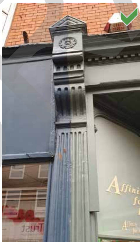
Treatment of original pilasters intended to separate shop fronts varying within adjacent shop frontages dependent upon which shop owner takes responsibility for the architectural element. The detail, if intact, should remain visible and not hidden in favour of bland over boarding matching inappropriate fascias.
