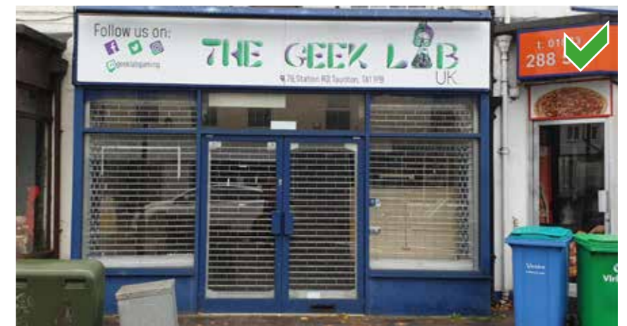
Internal grilles that provide visual connectivity to shop interior: preferable security option
