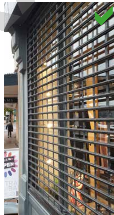
External security grilles set within the window frontage of a Grade II listed building, allowing visual access to shop window combined with successful way of securing a recessed entrance. The shop signage and fascia extends down in front of the blind box, but retains acceptable proportions in relation to the front elevation.
