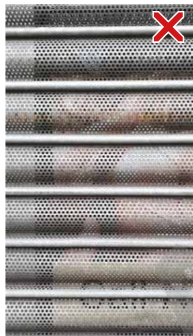
A fine mesh external shutter, with sufficient internal lighting allows the interior of the premises to remain visible after dark. By day however the appearance of this type is similar to a solid shutter.
