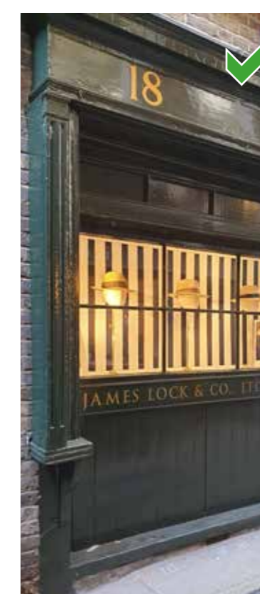
timber pilaster supporting fascia, with no capitol.
