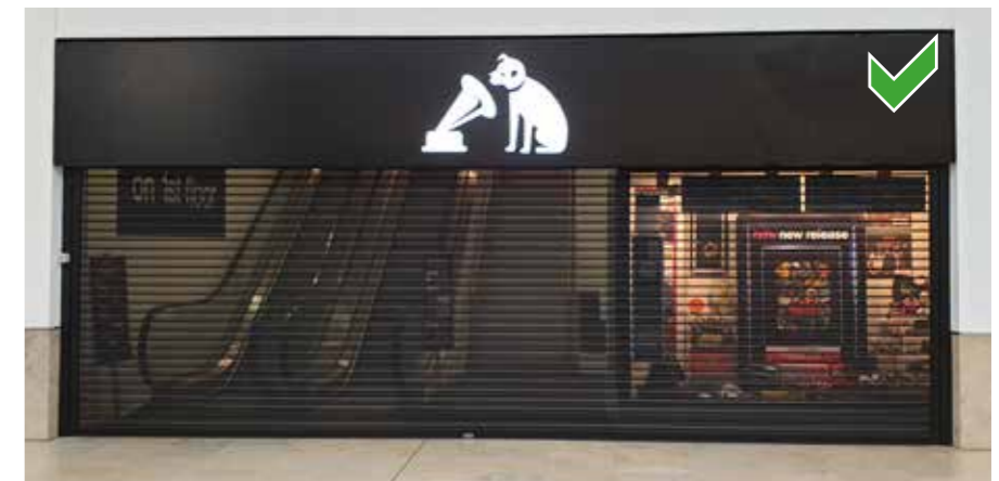
Internal lighting proves effective, illuminating window displays behind protective mesh grille - allowing illumination of the street scene and adding to the sense of a safer environment after dark: ideal security option
