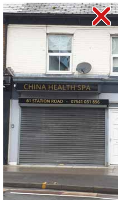
A fine mesh external shutter, with sufficient internal lighting allows the interior of the premises to remain visible after dark. By day however the appearance of this type is similar to a solid shutter.
